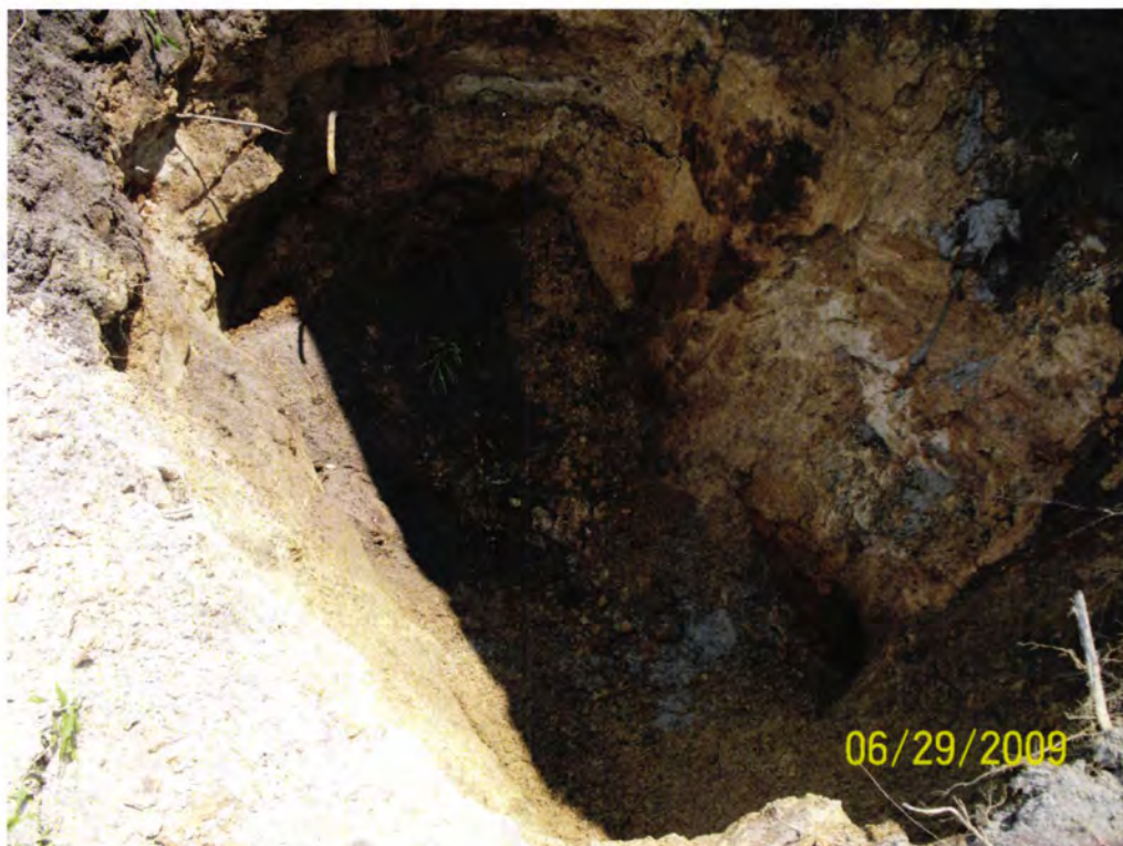
Picture 2: UST 480Laurelbay's excavation site.
